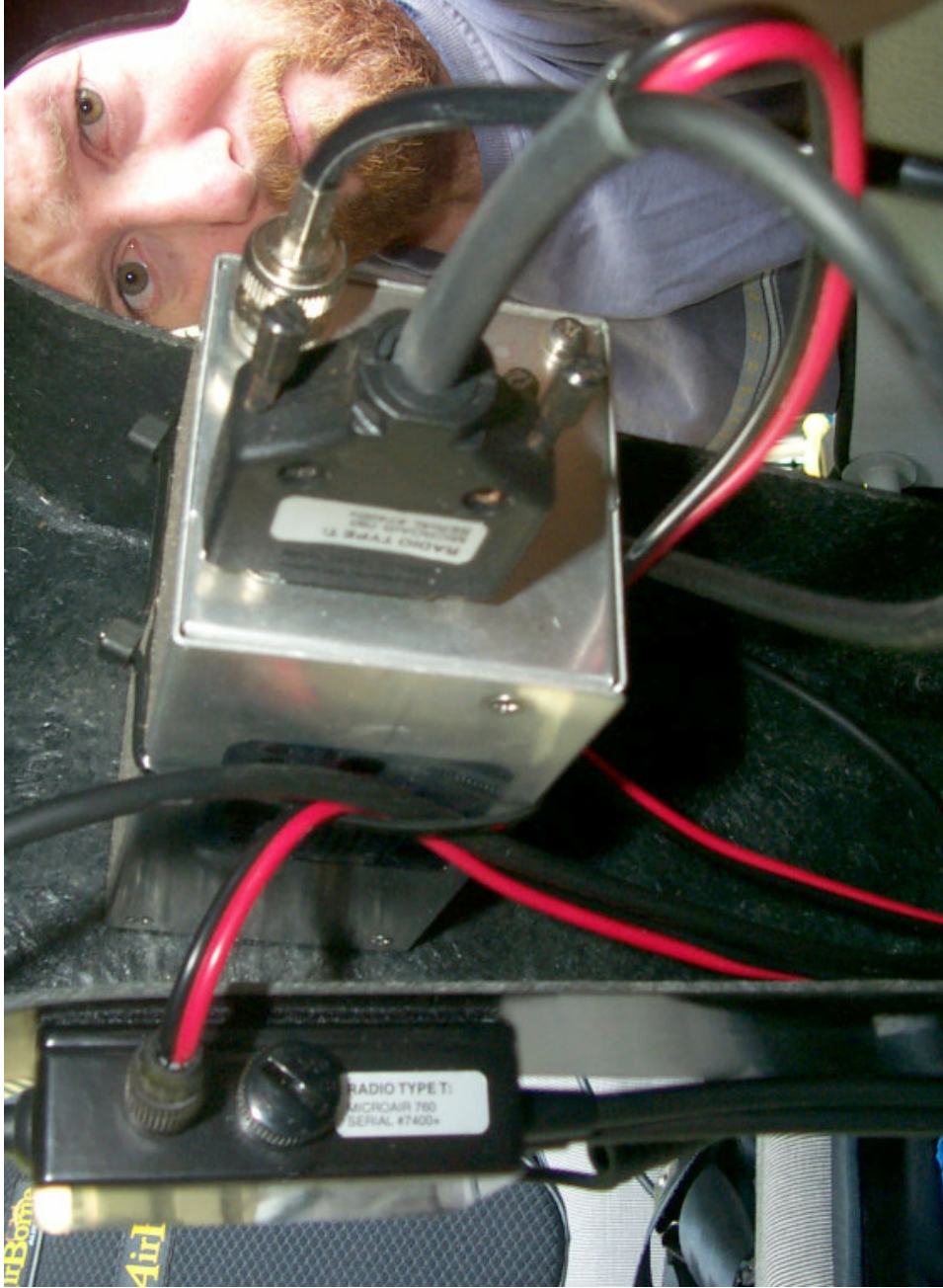
PHOTO SHOWS WIRE ROUTING AFTER INSTALL.
